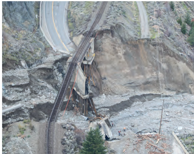
Figure 6 Damage to Highway 1 Tank Hill Underpass in British Columbia, Canada, due to extreme rain event in November 2021
