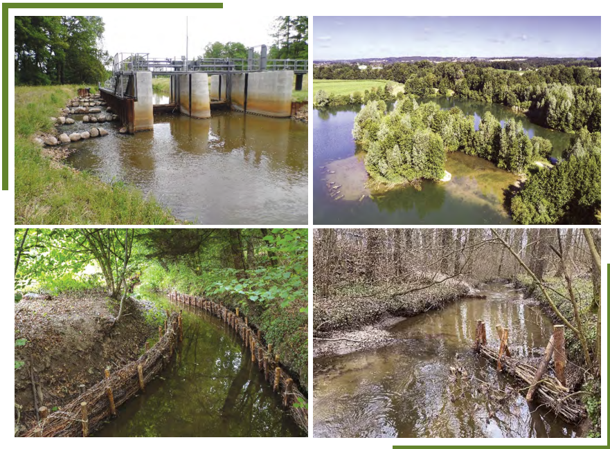
Figure 2: Examples for habitat development: mitigation of fish migration barriers by construction of a technical fish pass, creation of shallow bays in a gravel pit lake, structure enrichment and current diversion by installation of tree trunks and branches (clockwise from upper left; photo credits: S. Zahn, IfB (1) and F. Möllers, Anglerverband Niedersachsen (2-4))
