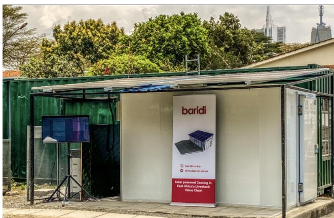
Figure 1: Unit 1 Solar-powered Chiller
