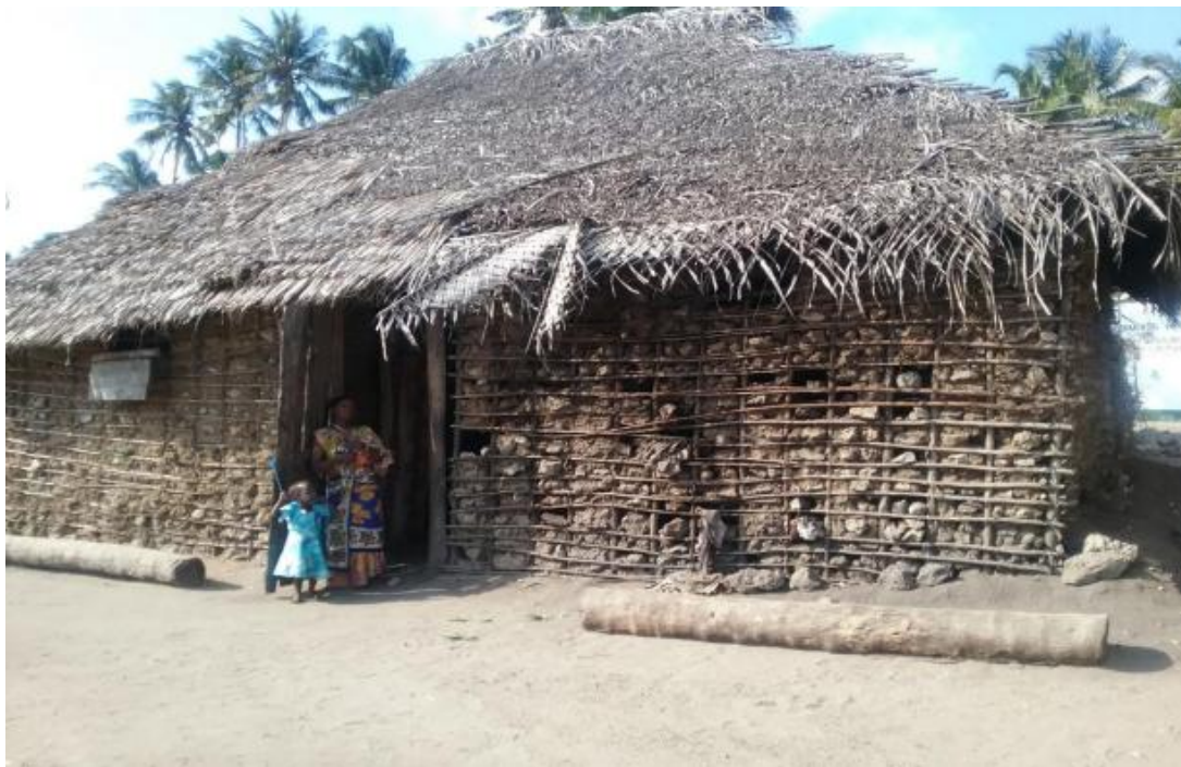
Plate 2. House showing the use of poles from mangroves for construction.
