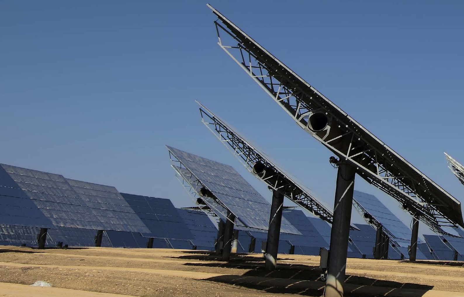
Mirrors and tower of the 11 megawatt PS10 (Planta Solar 10) operating near Seville, Spain. The world's first commercial concentrating solar tower power plant. © raulbaenacásado
